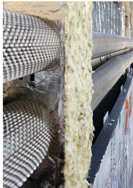
Firebreather® Cavity Barriers strategically installed at floor level to ensure optimal compartmentation of the facade, enhancing fire safety by preventing the spread of fire between floors.
